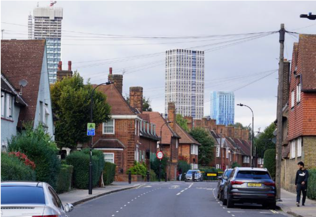
Figure 8: Tall Buildings Visible from within the Conservation Area
